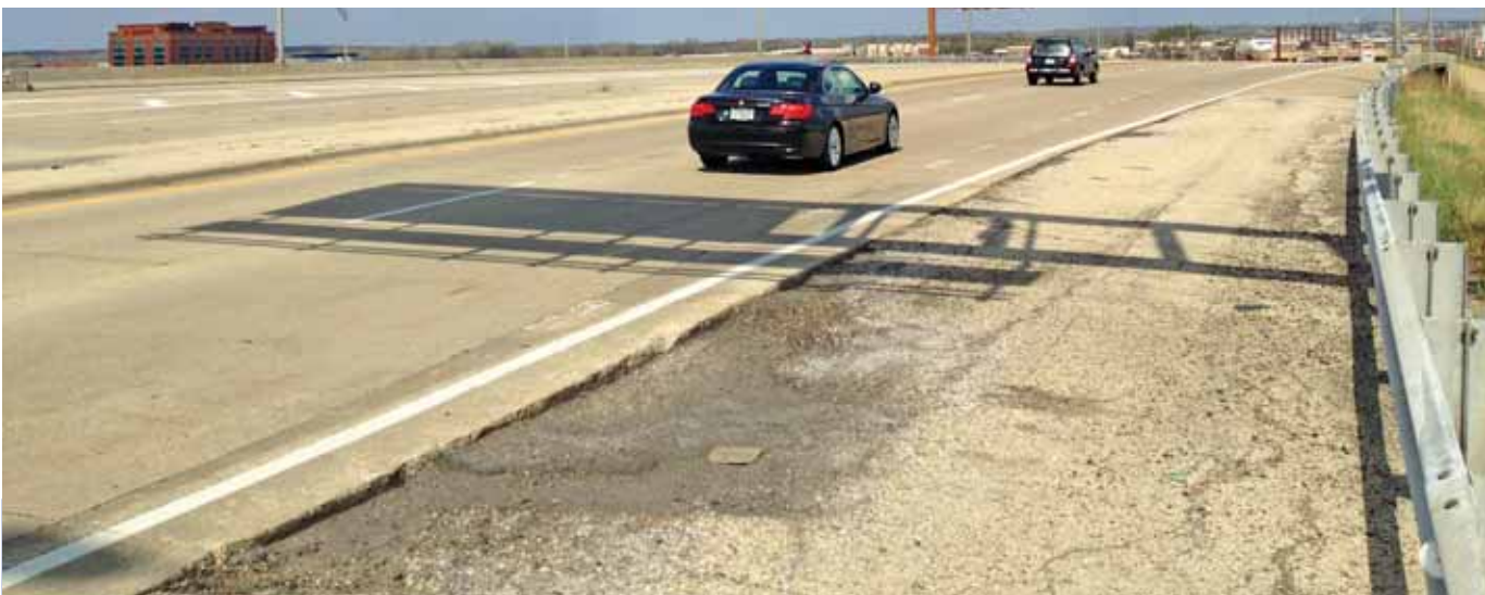
IDOT has established an annual dedicated line item to fund the deck-sealing program and has had success with letting contracts for deck sealing only within each of its nine districts. Contracts are advertised and let in the spring with application of the sealer in the summer.
