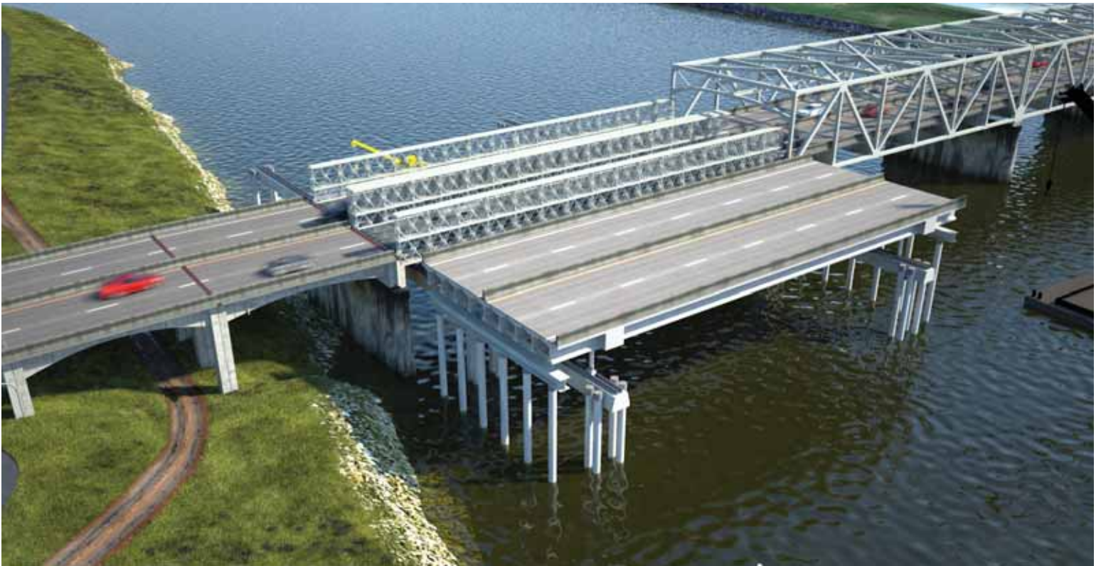
The winning bidder decided to go with a bulb-T lightweight concrete girder design for the permanent span.
