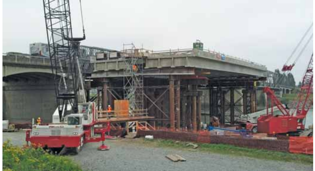
The girders have very wide top flanges, so the distance between each girder was 12 in. except in the center where crews were going to cast a median barrier, which required a 4-ft-wide closure pour.
