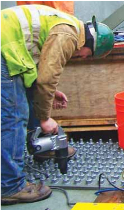
Rather than rely on the laborious method of tightening each nut so many turns to reach the steel's capacity, the crew installs each bolt with a shear gun.
