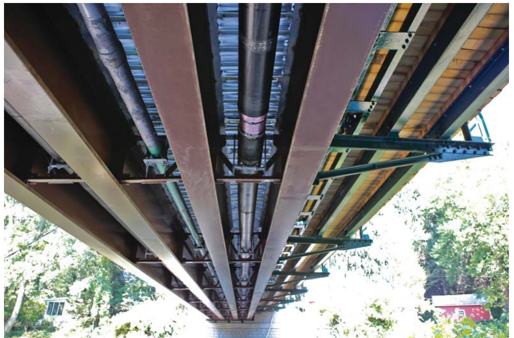
Below: The steel multigirder superstructure allowed the removal of weight restrictions while preserving the historic flavor of the original truss structure. Moreover, three bays carry water, sewer and gas lines between Cornell University and the Forest Home community.
