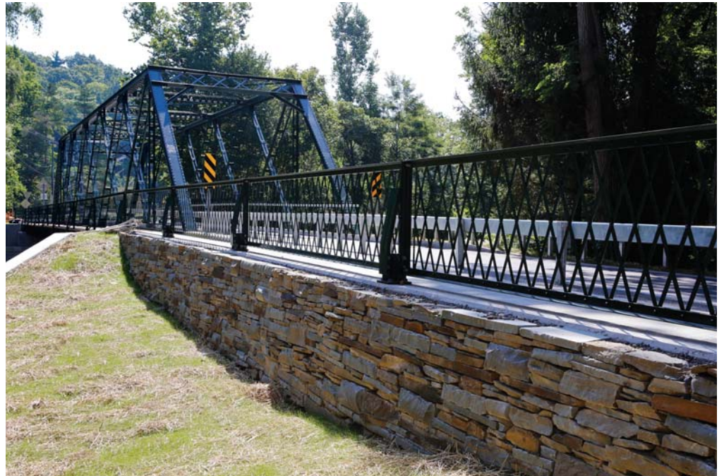
Above: The Ithica, N.Y., bridge is registered in the National Register of Historic Places; its original truss steel dates from the Model T era and had a 15-ton load restriction.
