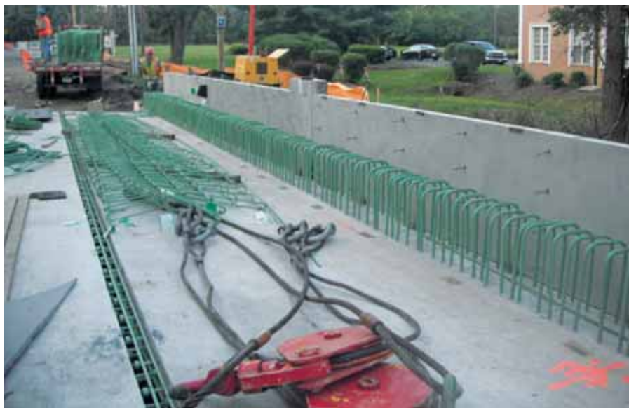
Four new 92-ft-long precast superstructure units consisting of dual steel-plate girder stringers in composite action with a reinforced high-performance concrete deck were installed atop new bearings. The longitudinal joints were filled with quick-setting cement.
