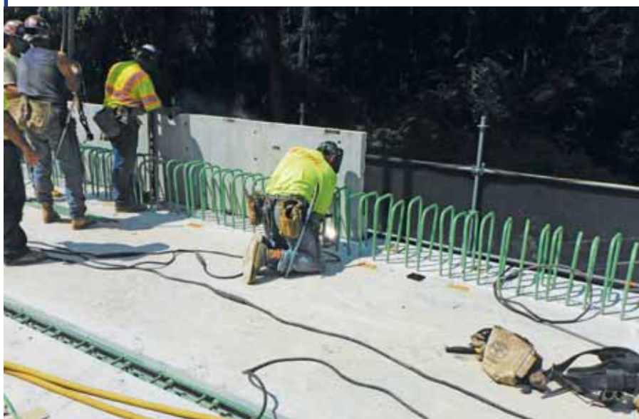
Four new 92-ft-long precast superstructure units consisting of dual steel-plate girder stringers in composite action with a reinforced high-performance concrete deck were installed atop new bearings. The longitudinal joints were filled with quick-setting cement.
