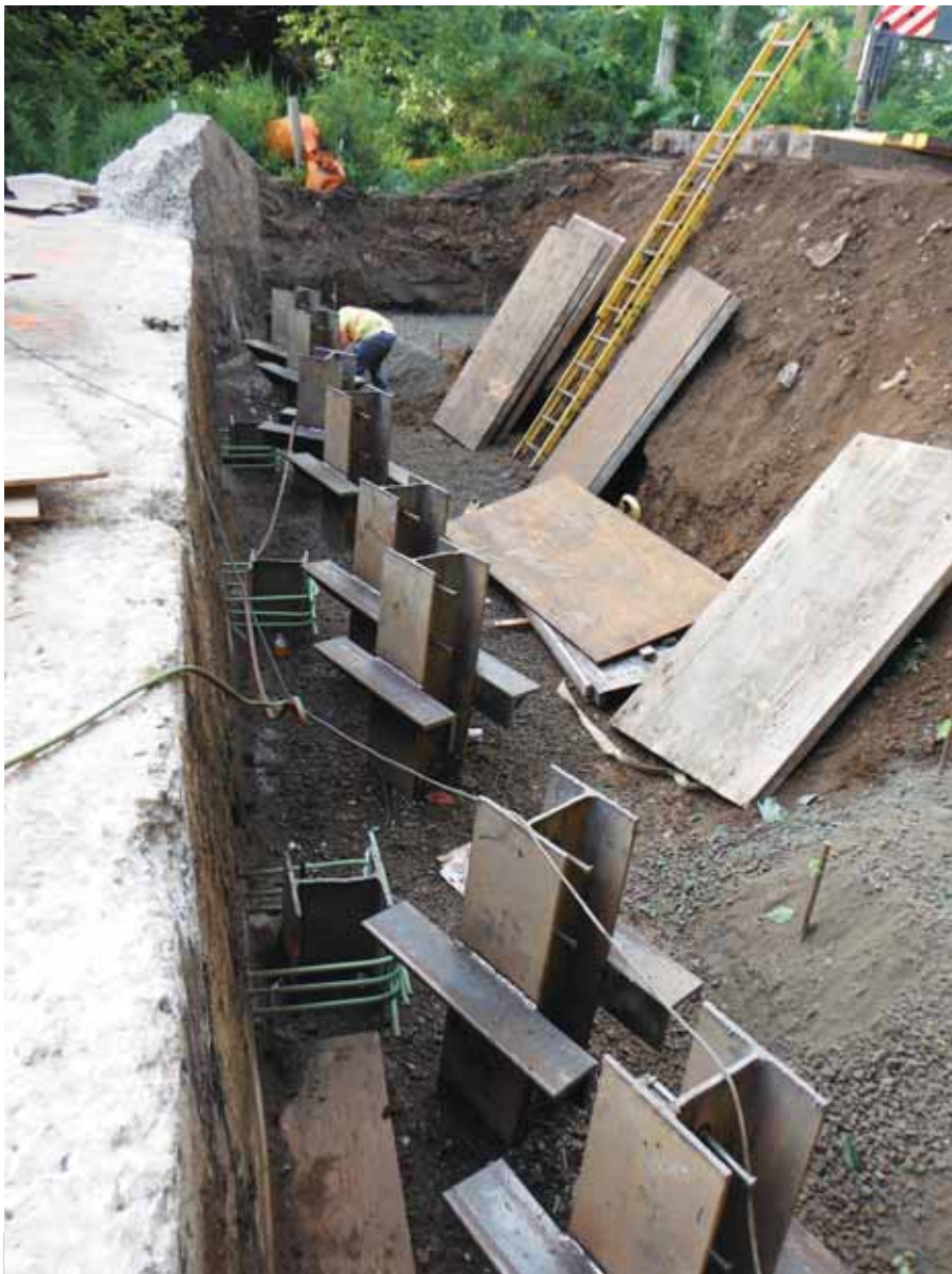
Construction staging was designed to keep all construction impacts within the footprint of the existing road and bridge. This resulted in no disturbance to the surrounding area.
