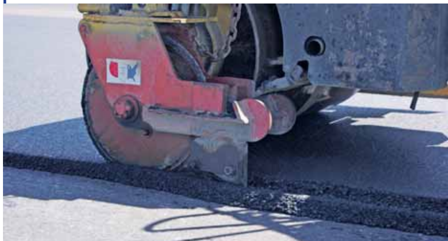
Below: The longitudinal joint down the middle of the NOLA track is cut by a special roller with a cutting wheel following behind the other rollers.
