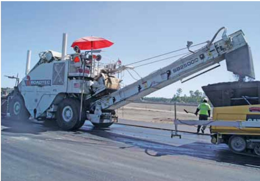
Barriere used a material transfer vehicle, skis and sensors to ensure the asphalt surface was smooth. With a 0.1-in. blanking band, they saw a profile index of 8.6 in. per mile.
