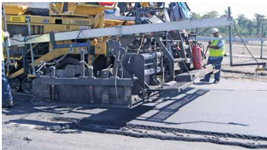
Above: The paving crew attempts to place the screed exactly where it was when it encountered a problem getting around a sharp corner.
