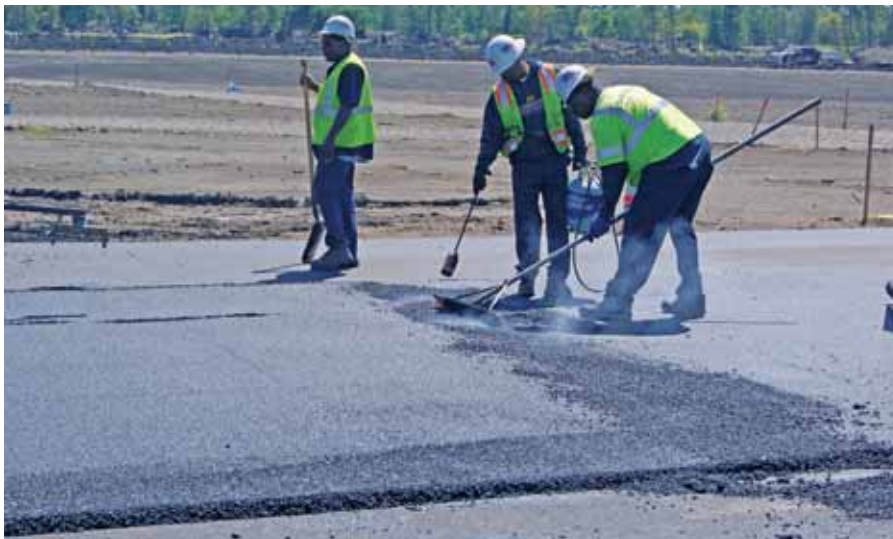
Workers heat and smooth a transverse joint by hand. The asphalt mix used at NOLA is a 5-in. pavement, put down in three lifts. The base course is 2 in. of a conventional Louisiana DOT mix, with 12.5-mm aggregate size and a 67-22 or 64-22 binder.
