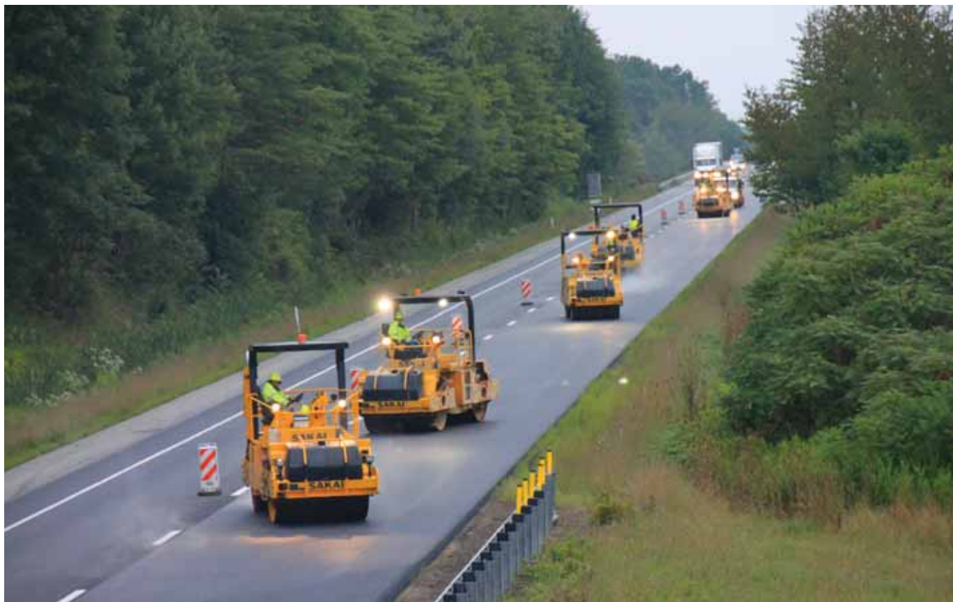
Four or five Sakai high-frequency rollers were used; the number of rollers was dependent upon the production schedule. The rolling pattern consisted of between five and seven vibratory passes per roller. The last roller in the paving train was operated primarily in the static mode. Whenever possible, all rollers would arc off the mat at the end of all passes onto a previously placed surface.
