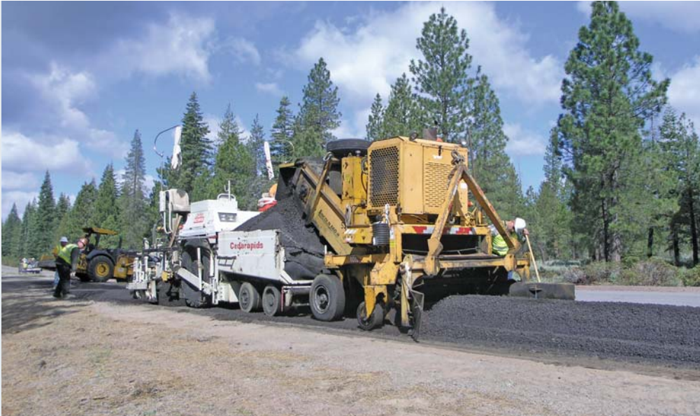
Far Left: A Wirtgen W 1900 was one of two cold mills tackling the 7-mile stretch of Mooney Road.
