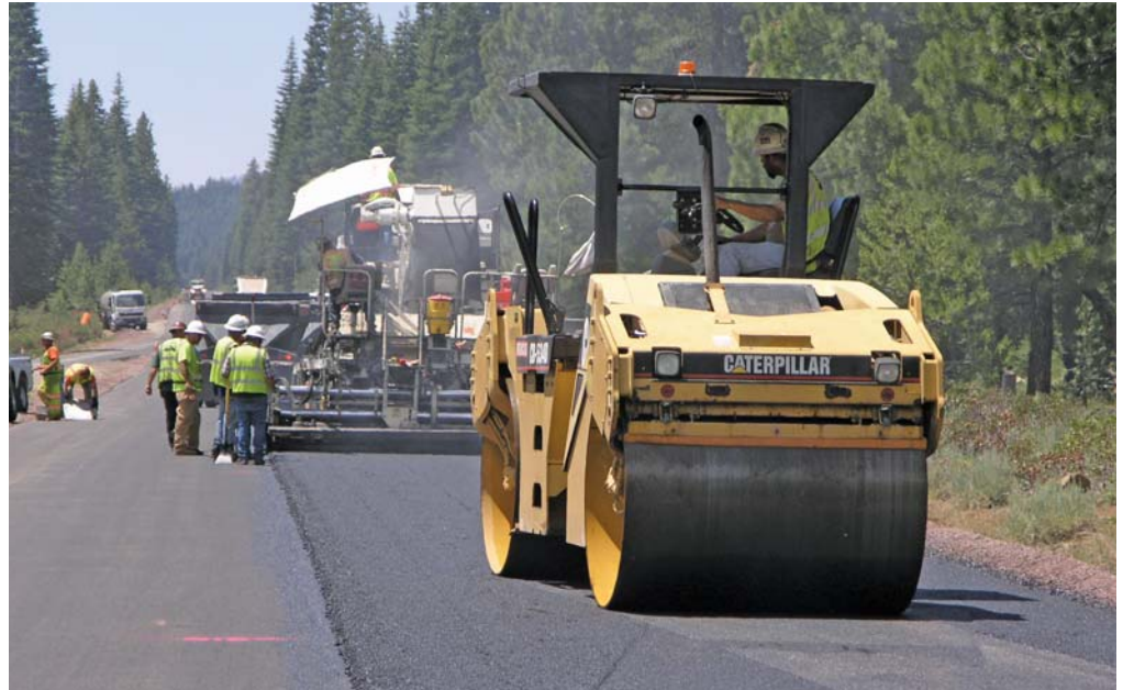
Two Caterpillar rollers were used for asphalt compaction on the Mooney Road project, allowing the project team to achieve 92% smoothness for an incentive bonus.
