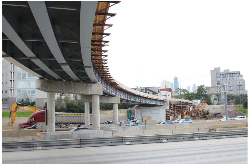
The new Ontario Street mainline ramp is a three-span continuous multigirder bridge that carries a single lane of traffic from westbound Ontario over the Kennedy Expressway.
