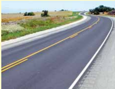
Norris Asphalt widened Highway 34 from 24 ft to 32 ft, adding a new 4-ft shoulder on each side of the roadway.
