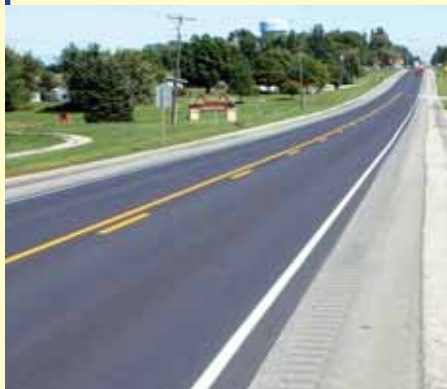
Norris Asphalt widened Highway 34 from 24 ft to 32 ft, adding a new 4-ft shoulder on each side of the roadway.
