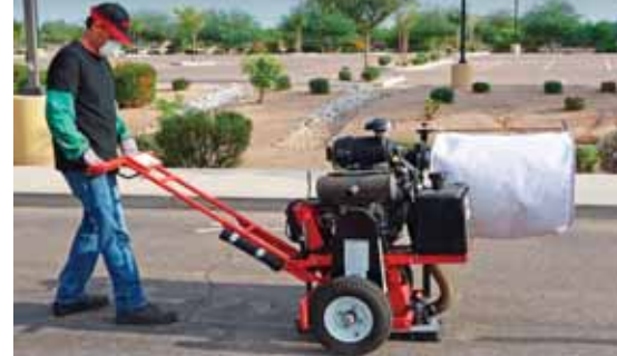
Crafcro routing with Crafcro crack-sealing has proven to last over 7 years 1
