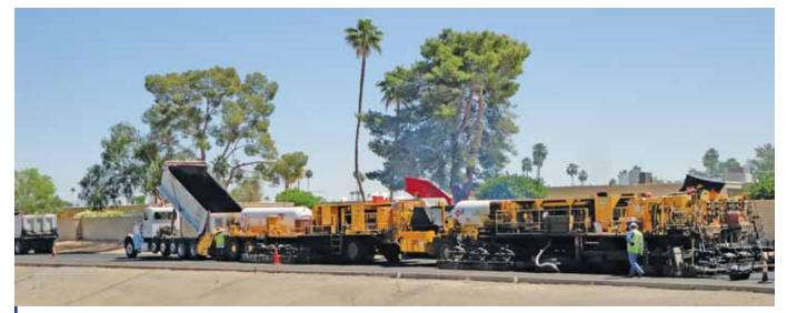
Cutler brought in its own paver. Going one lane at a time, the machine heated, scarified and recycled the top layer, refreshing it with new asphalt emulsion. While the recycled content is still hot (at least 200°F), an additional inch of fresh material is placed on top.
