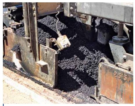
The paver can be augmented to any width needed via a series of pre-made, 1-ft extensions for the heating head, scarifying teeth row or the recycling auger. This adaptability allowed Cutler to set a new Arizona record with one pass of 18 ft.
