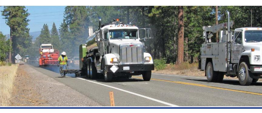
results with the added benefits of reducing smoke and emissions during the chip seal application. The pilot projects also evaluated the aggregate retention, aggregate embedment, raveling and resistance to reflective cracking.
