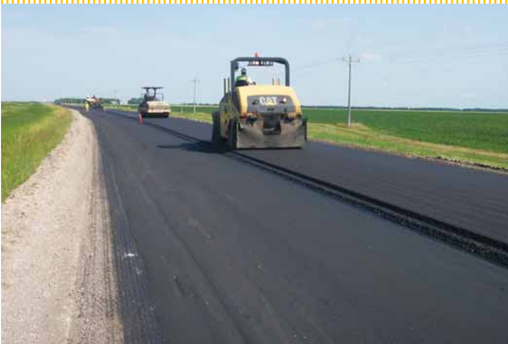
Knife River used Ingersoll Rand DD158 steel-drum rollers for intermediate and finish compaction after using a Cat 360 rubber-tire roller for the breakdown function and achieved 89% of the available bonus for smoothness and 98% of the available bonus for density.
