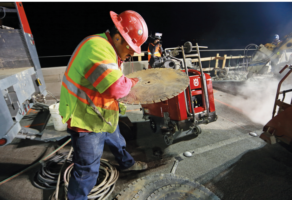
Workers completed the jacking operation and installed seismic joints with a full closure at Pier 31 on Labor Day. That was one of only two full closures of the bridge they needed.
