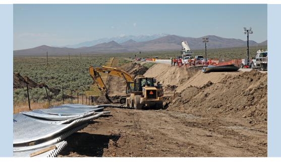
The underpasses on Rte. 93 are made of large corrugated metal spheres that pass under the roadway. Partial road closures were required during installation. Photo courtesy of NDOT.
