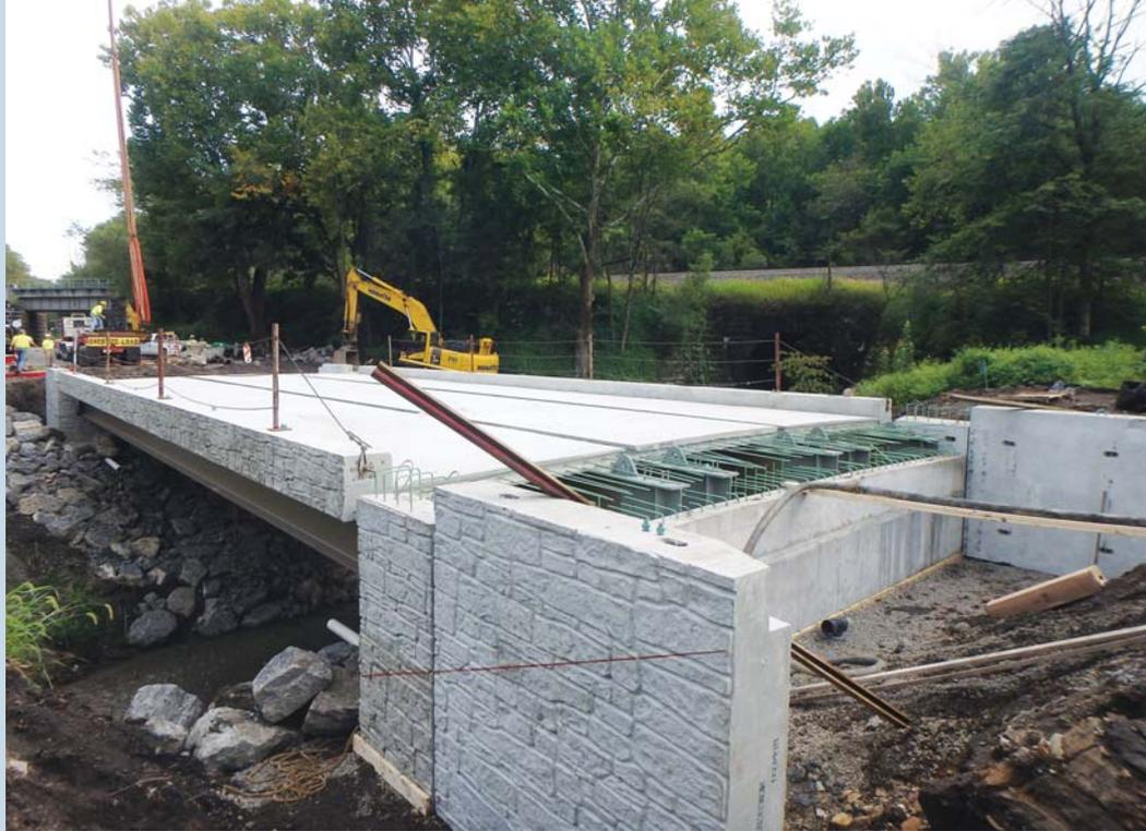
and the superstructure. This support was needed to allow construction to continue while the grout cured in the CMPs. The rolled steel beams were delivered to an off-site location where the reinforcement was tied and placed for the deck and barrier. Since the District's preference was to avoid precast deck panels, cast-in-place concrete was used. The beam/deck/barrier modules were delivered to the project site and connected using ultra high-performance concrete (UHPC).
