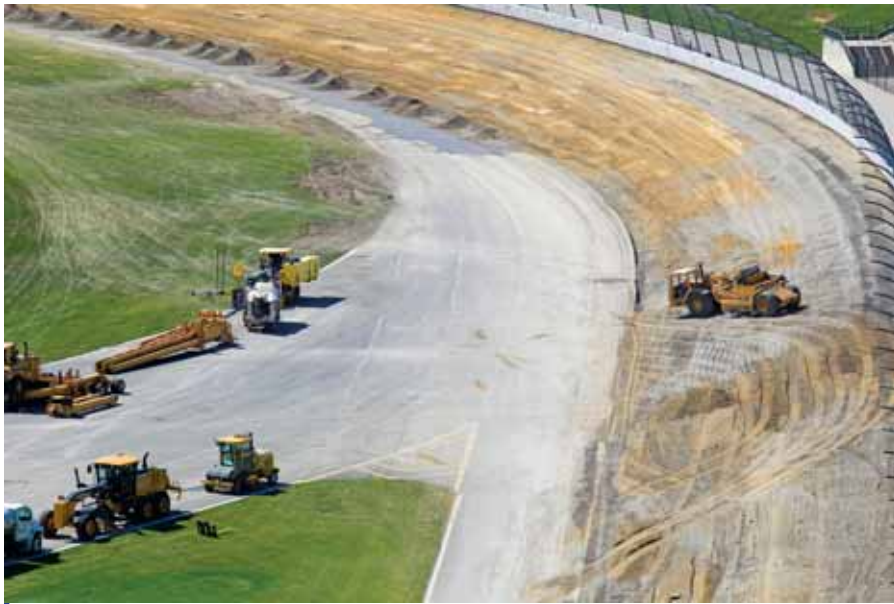
Caterpillar D6T and D6R dozers were cutting as much as 2 ft deep into material to establish the new slopes on the turns. The original plan was to push the bulk of dirt upward before a Caterpillar motor grader smooths out the surface.
