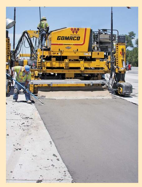
for us," Gough said. "We're doing a lot of paving with a 2% or more slope. The plow helps us keep the material where it needs to be. The Commander III is very capable of doing just about anything that needs to be done, and we're proving that on this project."
