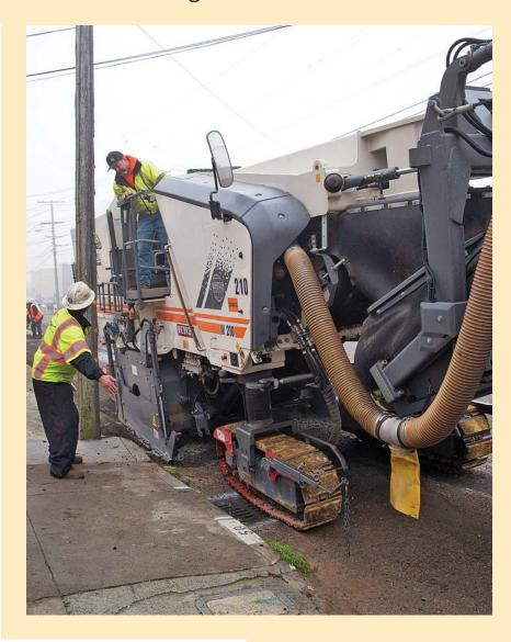
"Once you finish a cut, you turn off automatic, pushing one button, and the machine just lifts up out of the cut all by itself," Allende said. "It's one less thing for the operator to think about."
