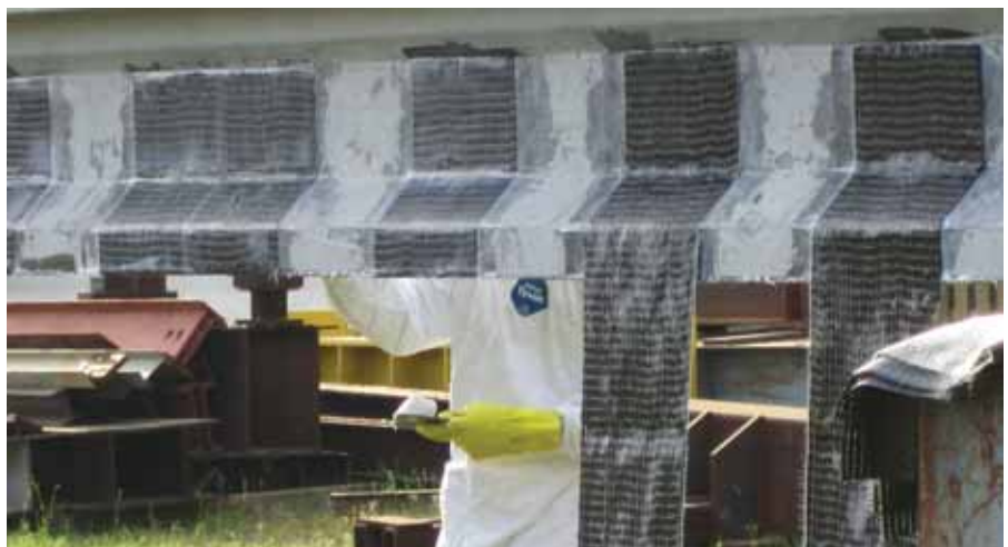
The half-scale and full-scale girders had a variety of repair configurations with several numbers of CFRP layers and with different spacing for the U-wraps. The full-scale PSC girders statically tested were arranged in a similar manner to the half-scale specimens.
