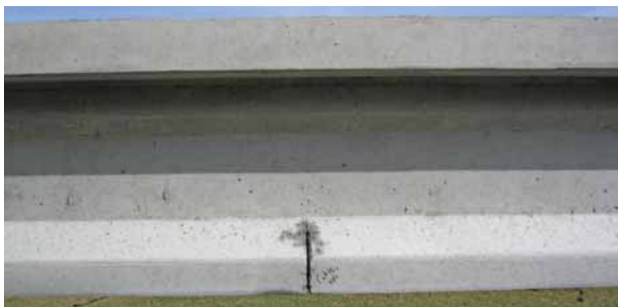
The lateral damage simulation for each girder was achieved by sawing through the concrete of the bottom flange and slicing through one of the prestressing strands.
