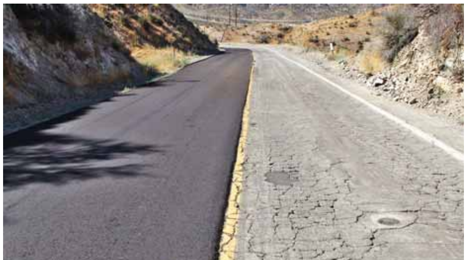
With an average pavement condition index (PCI) of 47, the road seriously needed to be rehabilitated, according to Imelda Diaz, P.E., with the Los Angeles County Department of Public Works and head of the county's pavement-management unit.
