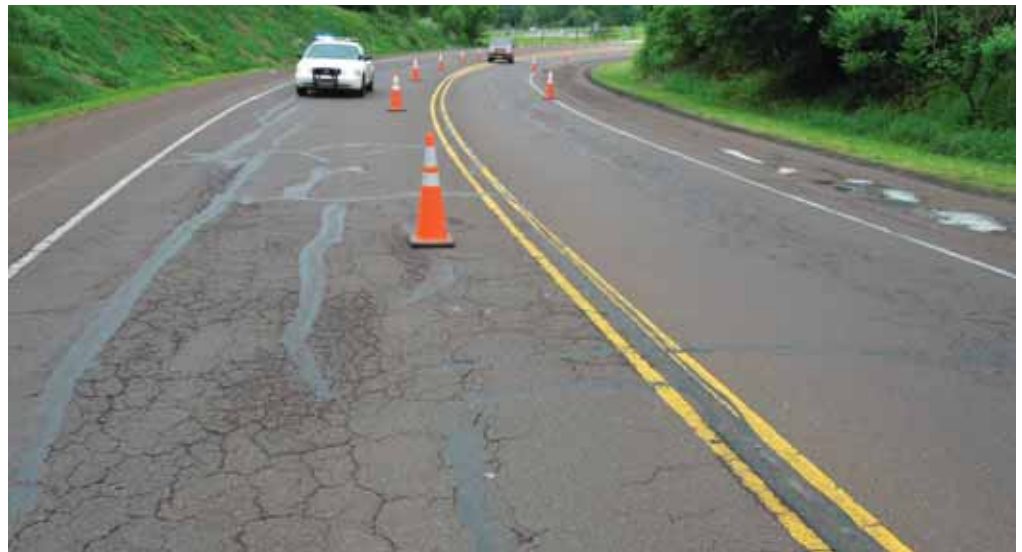
Above: The ramps and mainline pavement of Rte. 202 that led motorists to and from the Delaware River Bridge looked like it might require double the work. Alligator cracking and areas of settlement started saturating the area, especially on the ramps on the Pennsylvania side of the span.
