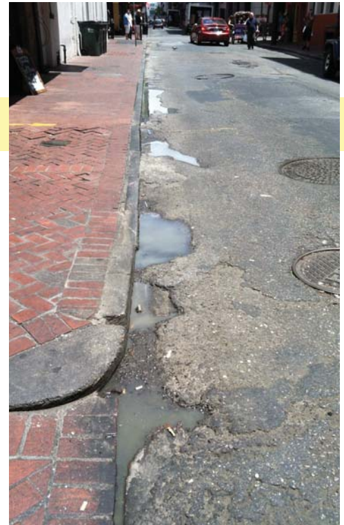
Iberville Street was restored from a crumbling state of patchwork and potholes that caused significant standing water and poor drainage.
