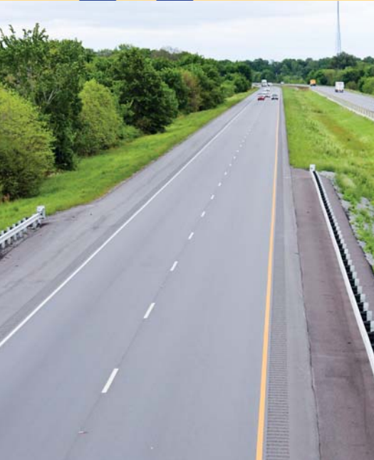
413,000 tons of asphalt were used to bring the 10.3-mile section of I-40 up a full foot.
