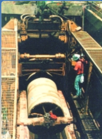
Using 25 tons of force to push 4,700 feet of 48-inch pipe in live flow.
