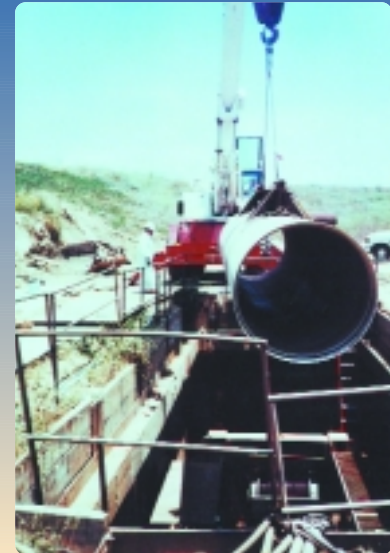
The lightweight pipe being lifted with a small mobile crane.
