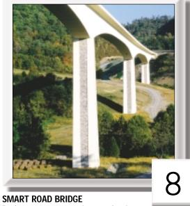
Few have seen a more attractive research project. The Smart Road Bridge, near Blacksburg, Va., was built to functionally support the state's Smart Road transportation research project. The state's tallest bridge—175 ft above the valley floor—is 2,000 ft long and features cantilever construction with cast-in-place segments and concrete-embedded, post-tensioned steel cable. Total cost: \$17.4 million.
