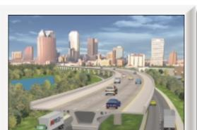
BRANDON PARKWAY Tampa, Fla., has tomorrow in sight. The Brandon Parkway is the future of highway expansion. This elevated structure will be a precast concrete segmental box girder bridge with precast segmental piers. Total
