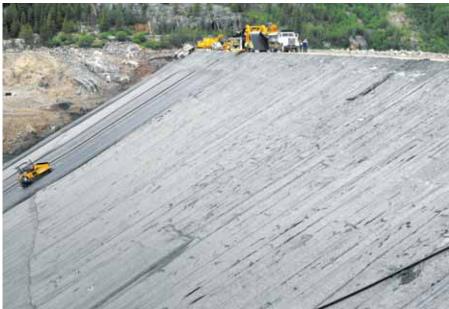
To properly place and compact the asphalt, large pieces of equipment, including a paver and rollers, were secured with cables attached to portable winches that allowed the equipment to be either lowered from the top of the dam or raised up the face.
