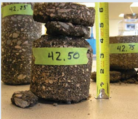
Severe moisture damage in intermediate layers.
