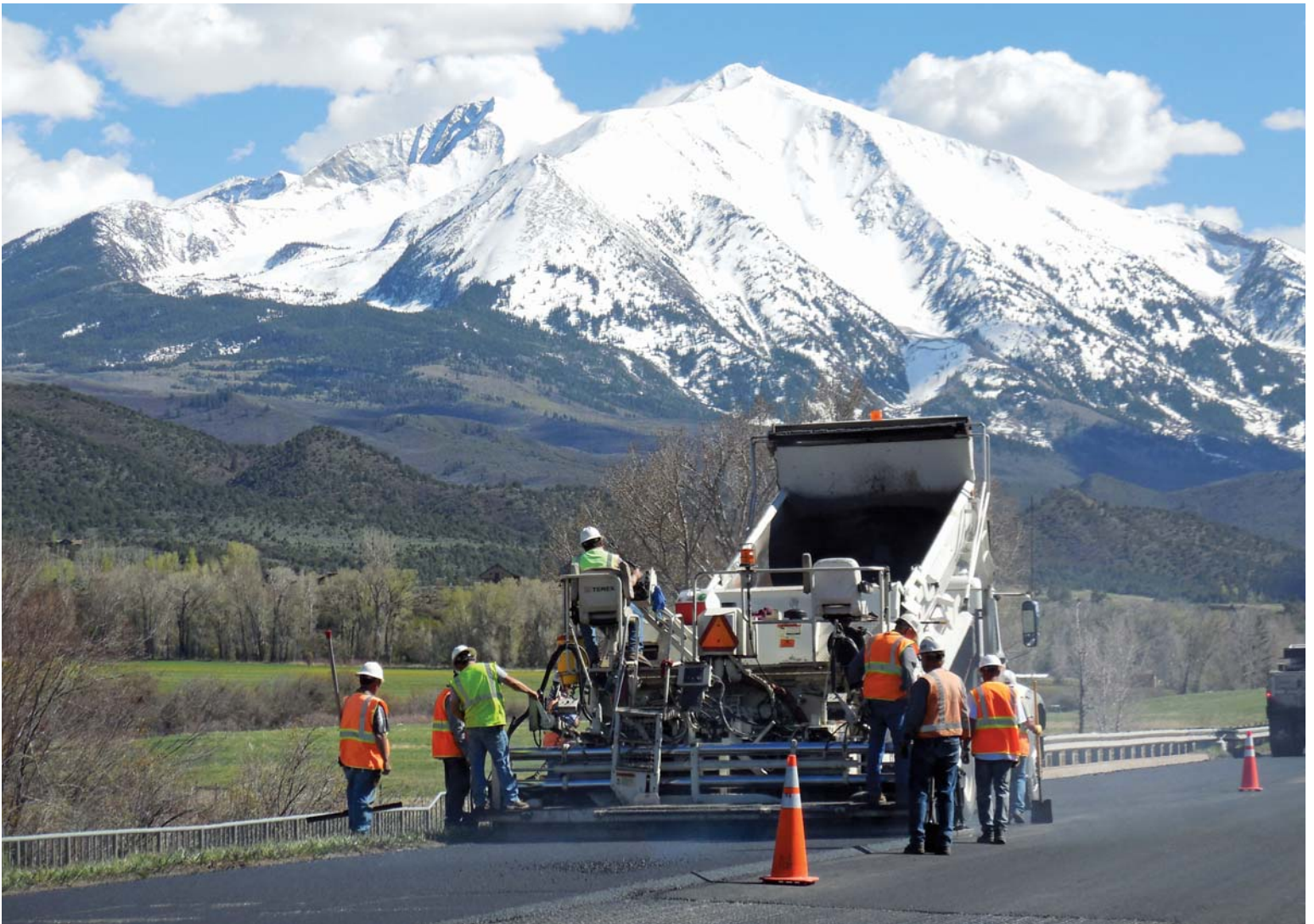
The Superpave mix employed on SH 133 contained 97% RAP. The average asphalt content was 6.6% and the contractor used a PG 58-28 binder.
