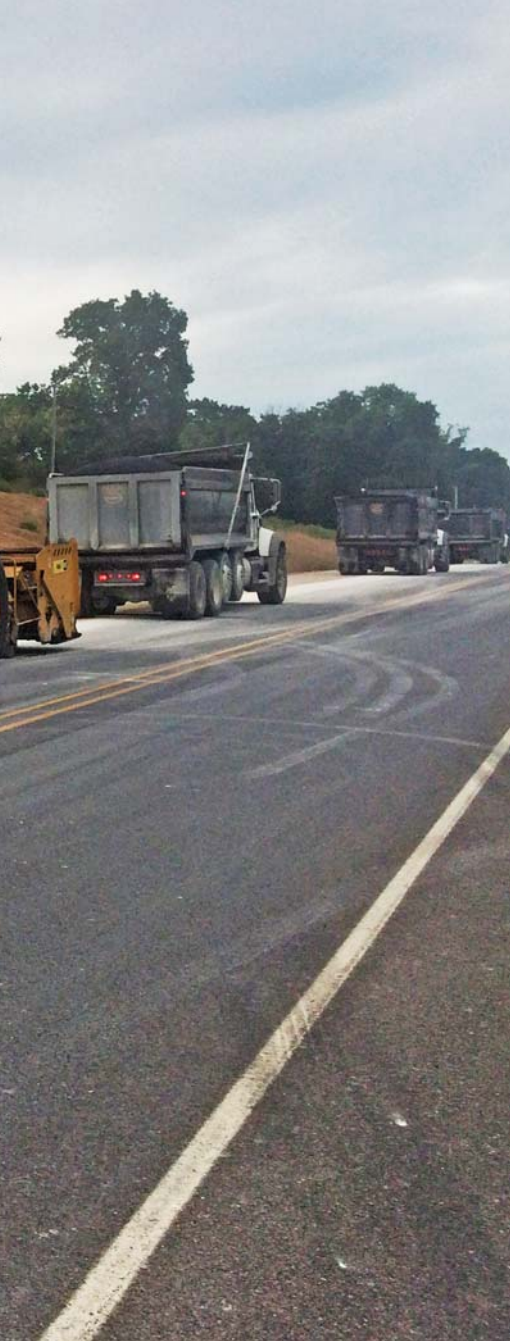
The two-year Highway 62 project resulted in one of the lowest profile indices in Arkansas—and is one of the state's smoothest roads.
