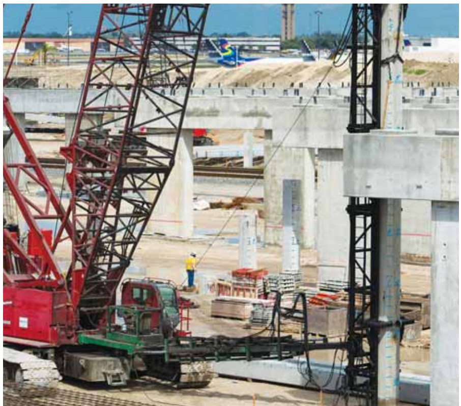
The taxiway will be mainly supported by cast-in-place, 3-ft x 10-ft piers—about 90 in all. Due to the soil conditions, concrete piles are being driven down to varying depths.
