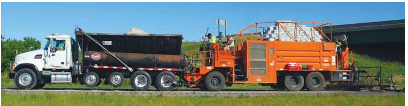
The continuous microsurfacing paver used by the Iowa DOT is set up with tanks for polymer-modified emulsion, water, aggregate, cement and an additive used to control the set. The trucks that support the paver will back in front of the paver to bring additional emulsion, water and aggregate to the machine. Photo courtesy of BASF Corp.
