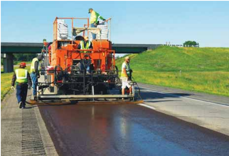
That microsurfacing can be used for both high-level interstate pavements as well as residential streets is a testament to their utility. Microsurfacing mixes are engineered products that use high-performance materials. Photo courtesy of BASF Corp.
