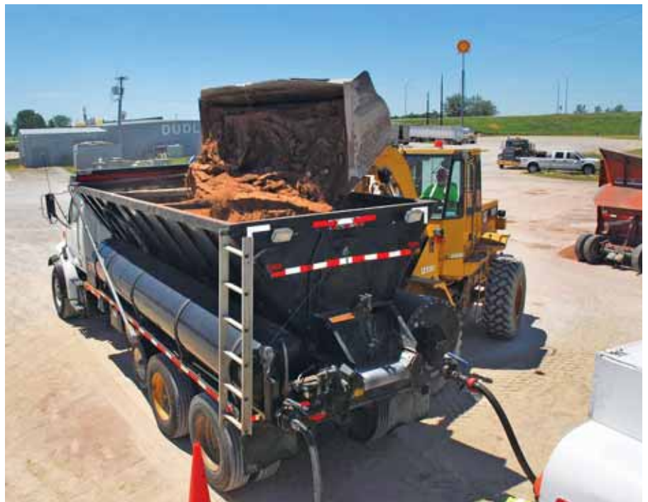
Microsurfacing was applied on I-35 in 2011 and again on a second project in spring 2012. The 2012 work—near Latimer in the north-central part of the state—was placed by Sta-Bilt Construction Co. Inc., Harlan, Iowa. Photo courtesy of BASF Corp.
