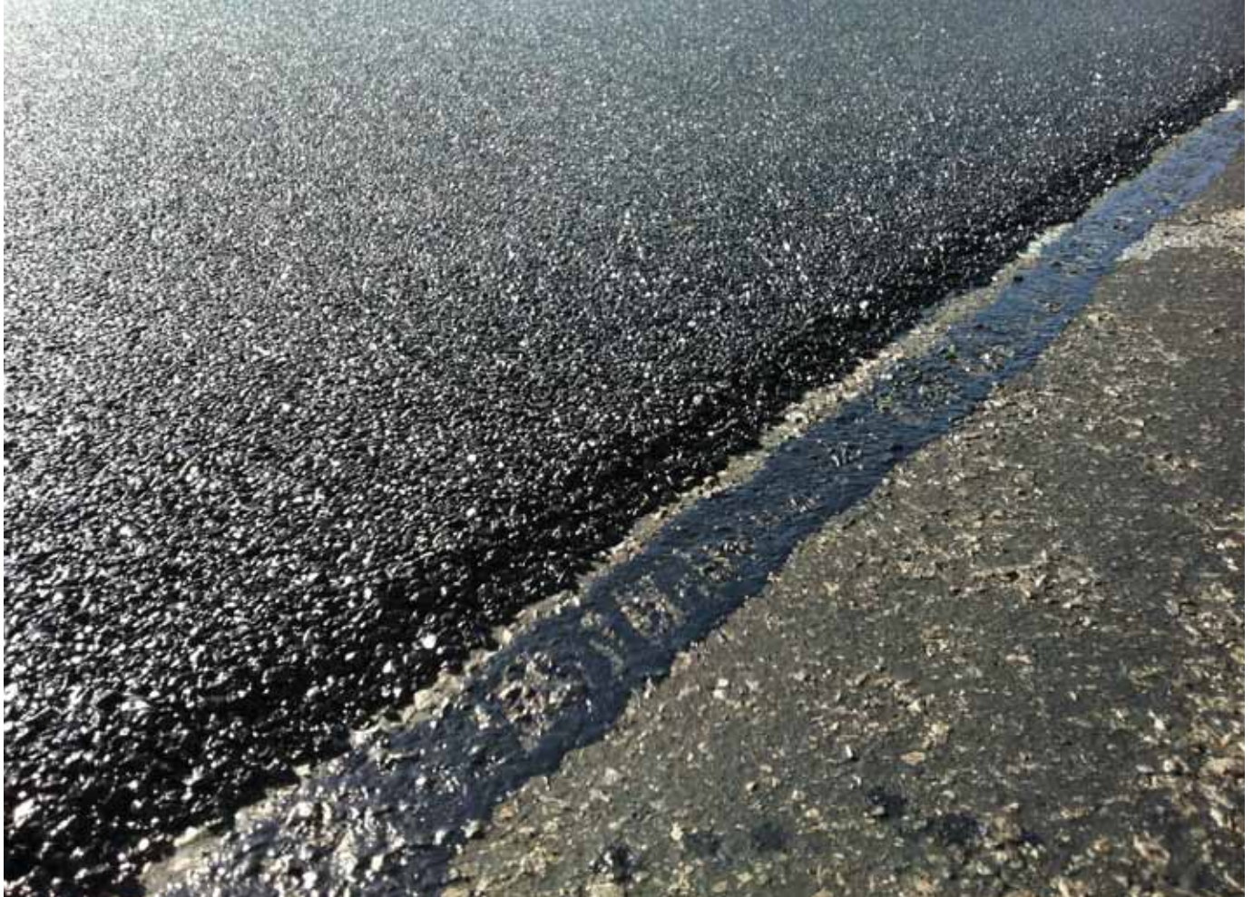
Thin lifts are susceptible to rapid cooling. During one project, researchers recorded mat temperatures during compaction.
