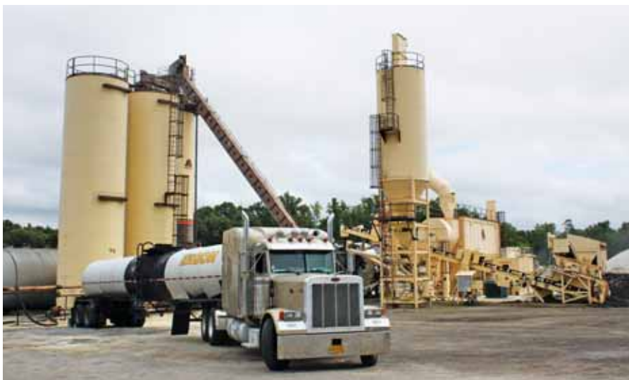
Three DOTs are sponsoring four sections as a Green Group, which will compare the performance and structural responses of four test sections that combine high-recycled-content mixtures with perpetual pavement design principles.
