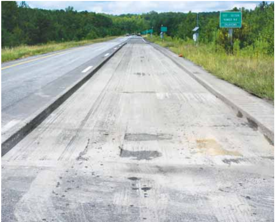
On Aug. 17, 2010, crews removed the top 5 1/4 in. of existing N8 pavement and replaced this with HiMA mix. Truck traffic resumed, and NCAT continued collecting data.
