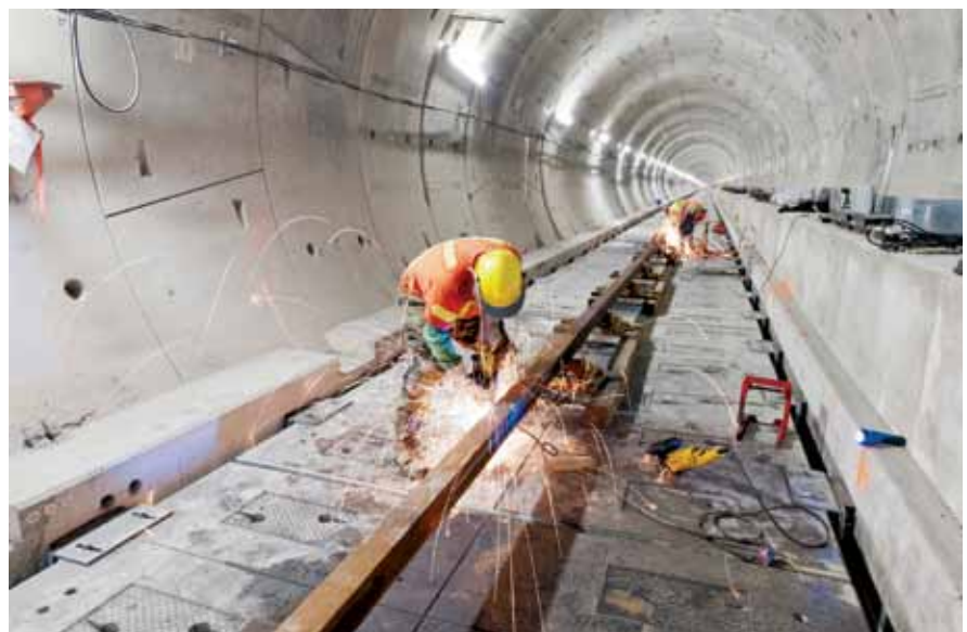
Workers welding rail in the new tunnels.
