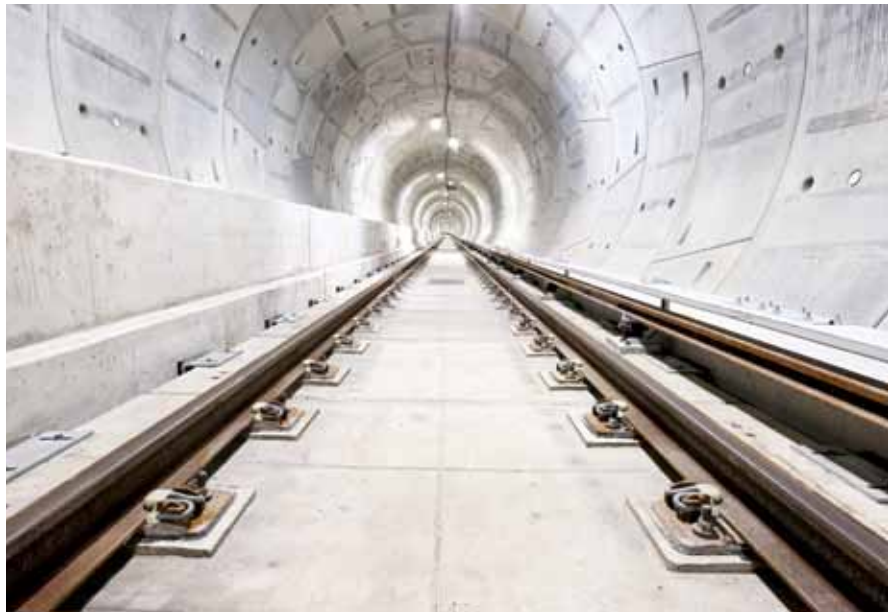
Completed track between Sheppard West and Downsview Park Stations.
